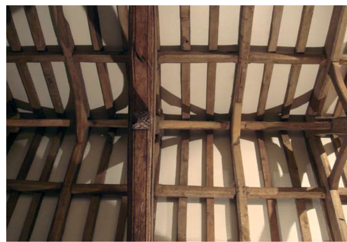
Tudor period roof timbers
